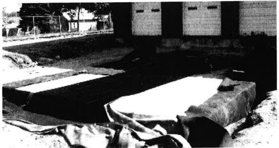
Rainwater harvesting system during construction (photo from Fox Valley Park District)
